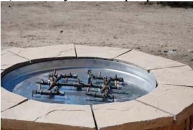
2) Apply lava rock ONLY deep enough to cover burner and pan less than 1” below crossfire burner jets.
