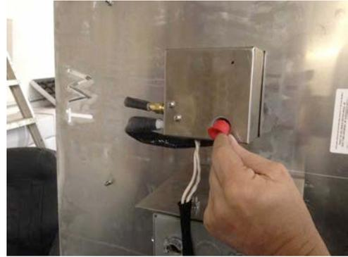
4. Apply pipe dope to the gas stub and compression fitting and thread to AWEIS control box onto the gas riser as shown in the photo at right.
