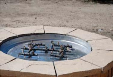
2) Fill Pan with glass. Cover Burner with 1/8 to .” of glass. Do not over fill with glass. All LP installations must be checked for back pressure with media installed. Failure to do so may result in personal injury or property damage.
