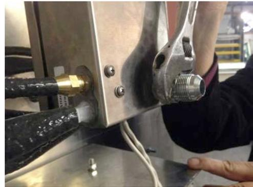
5. Attach flex line coming from key or service valve to compression fitting attached to AWEIS control box.
